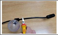
(a). Cut off end of line terminator leaving enough cable to allow re termination.
